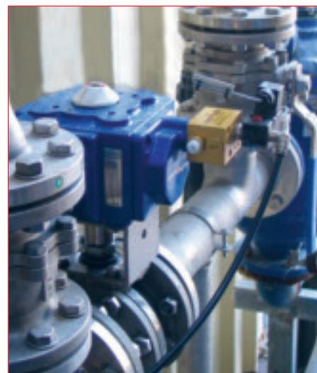
Habonim's IMPACT(™) increases closing torque on spring-return actuators.
