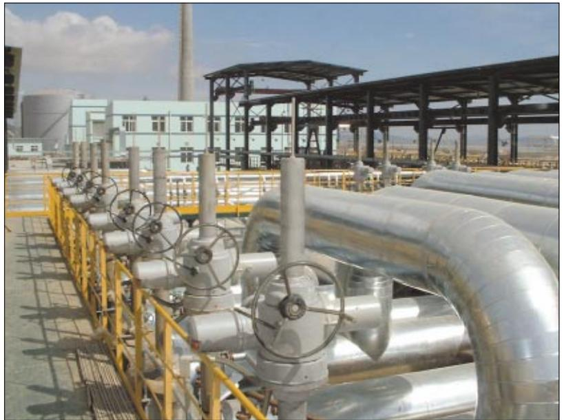
Rotork IQ90 valve actuators installed on a large Chinese tank farm manifold.
