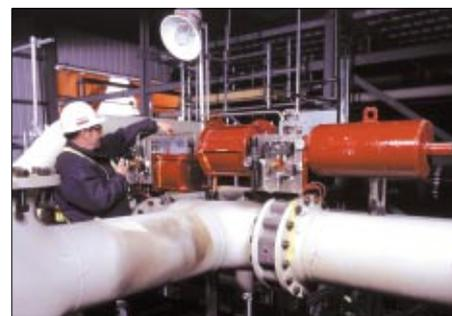
**GP range quarter-turn failsafe pneumatic actuators at the Cold Lake oil sands facility.**
