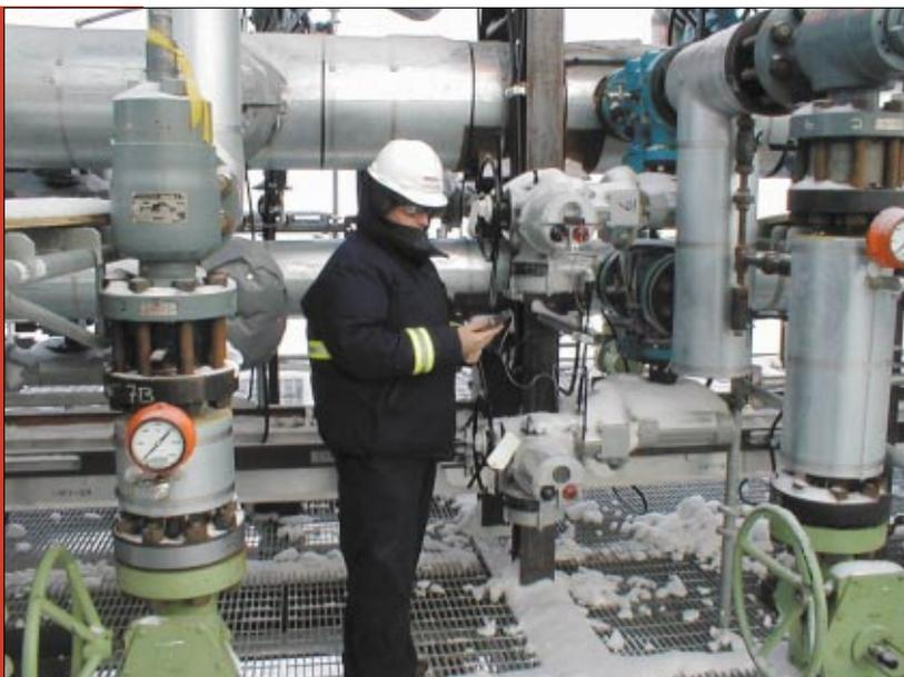
Non-intrusive IQ actuators have been installed in the freezing conditions of BP Borealis in Alaska.
