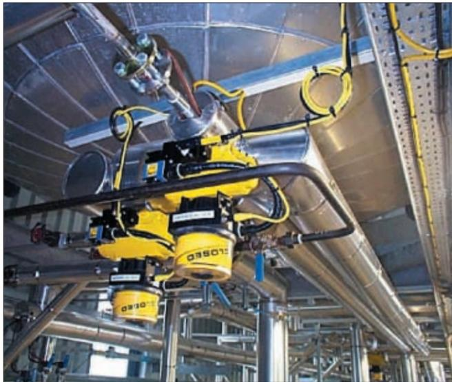
To meet Croda Universal's requirement of enhanced plant wide control, an integral package was put together comprising Hytork XL actuators, AS-i switch boxes and Hytork CATS (Clean Air to Spring) Solenoids.
