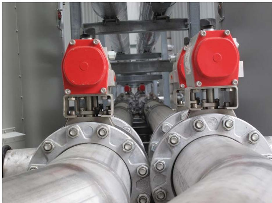
For application specific requirements the Series 98 offers additional options of extended travel stops, manual overrides and a hydraulic damper which is used for fast valve stroke applications. Engineered for efficiency, the compact design of the Series 98 generates output torques ranging from 10,600 to 885,000 in-lb (1,200 to 100,000 Nm).
