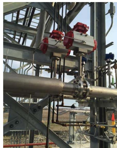
*Bray fully automated valve solutions operating in a cryogenic application.*
