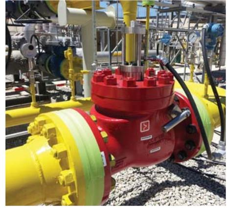
Rupture Pin's Model JA Pressure Isolation Valve.
