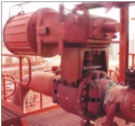
A 12" (300 mm) ASME Class 600 titanium autoclave discharge isolation valve used in nickel mining. Similar Velan Securaseal Metal-Seated Ball Valves are used for many of the mining industry's most erosive and corrosive applications around the world.
