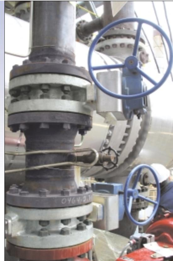
A double block and bleed set-up, incorporating 12" ASME Class 300 Stainless Steel Torqseal Triple-Offset Butterfly Valves on hydrogen service at 500 psi/480°C.
