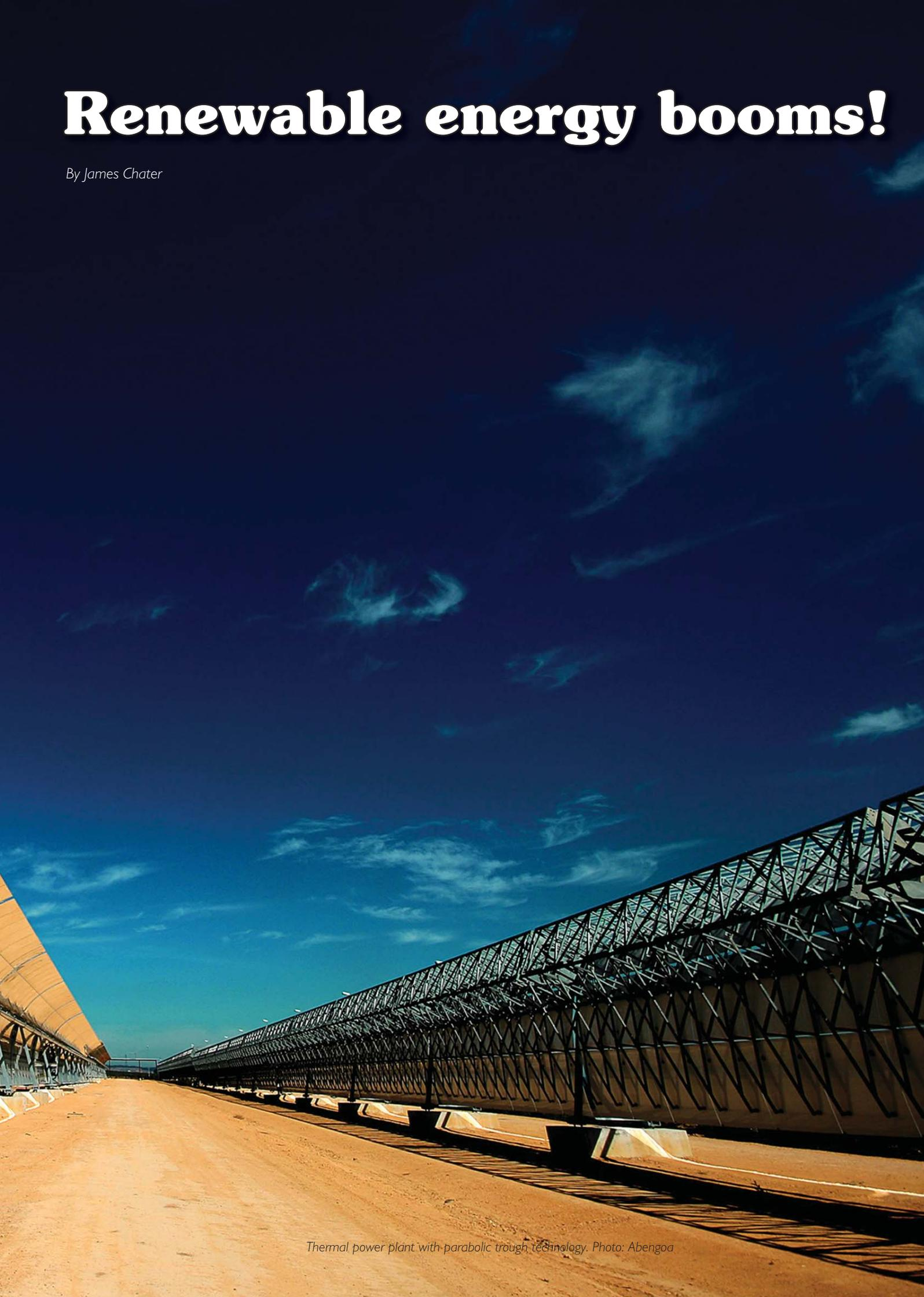
Thermal power plant with parabolic trough technology. Photo: Abengoa
