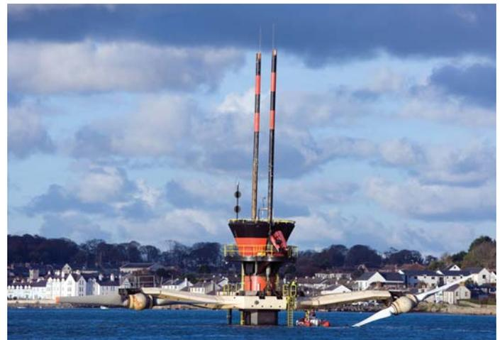
The SeaGen installation in the strait of Strangford Lough, Northern Ireland, uses tidal forces to generate electricity with the aid of two axial-flow turbines with a combined capacity of 1.2 MW. Two underwater rotors attached to a tower structure drive the marine current turbine. The twin rotors turn with the tidal current and optimally track the flow thanks to their 180-degree-pitch blades. Photo: Siemens
