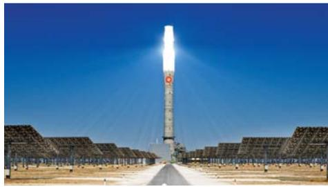
Gemasolar plant, owned by Torresol Energy. Photo © Torresol Energy Investments, S.A. Heliosdats (turning mirrors) reflect the sun's rays onto a receiver on the tower.
