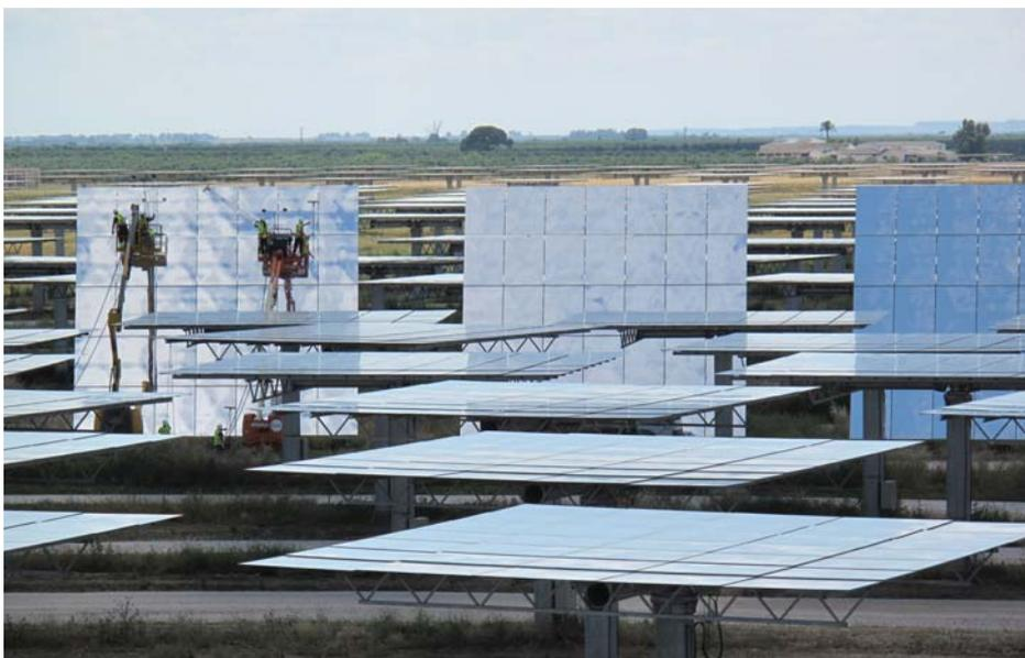
Figure 2: Cleaning of the heliostats at Gemasolar.
