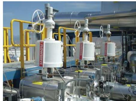
Figure 3: Flowserve control valves in molten salts service in a solar power plant at Andasol.
