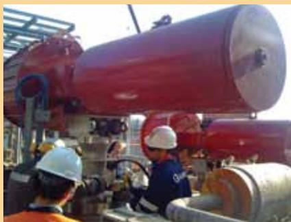
EuroLoop will be the world's largest research and test site for the calibration, verification and type testing of industrial flow meters and for the performance of industrial experiments involving process technologies and flow. The two closed-loop calibration circuits – one for liquid and one for gas – are fully automated, utilising Rotork RC Range pneumatic actuators, IQPro electric actuators and Pakscan P3 two-wire digital control.
