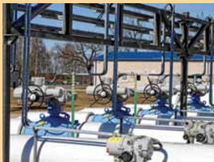
Rotork's CVA electric control valve actuator has been selected by the El Paso Exploration and Production Company in Wyoming, USA for water flooding – a method of secondary recovery in which water is injected into the reservoir formation to displace residual oil. The CVA's configurable failsafe capability, unlimited modulating ability, compact size and Bluetooth communication technology have contributed to the decision to install the actuators at five oil field well sites.
