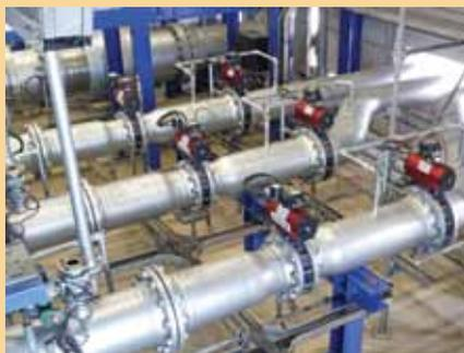
Underground gas storage facilities in Latvia are being developed and upgraded to secure the supply of natural gas to Baltic countries. At the Incukalna plant over 300 Rotork IQPro electric actuators are installed to operate ball valves controlling gas receiving and injection into storage wells. Modulating versions of the IQPro actuators are also installed in the site's metering plant.
